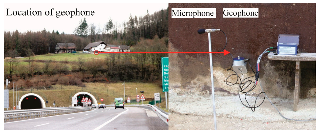
Figure 3. Facility where the monitoring was performed.
