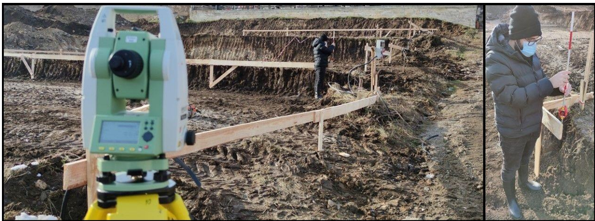
Figure 10. Batter boards survey.
