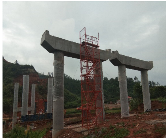
Figure 5. Field photograph of the test pier.
