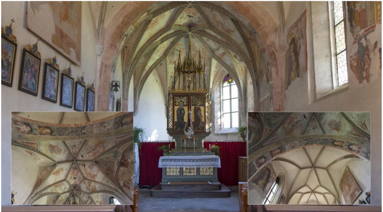
Figure 3. The vaulted system of the church. Source: F. Dalpiaz.
