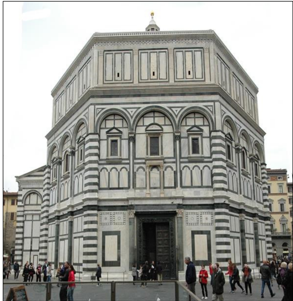
Figure 1. Saint John Baptistery in Florence (Italy), south façade cladded in white and dark marble according to the Tuscan Dichromic.
