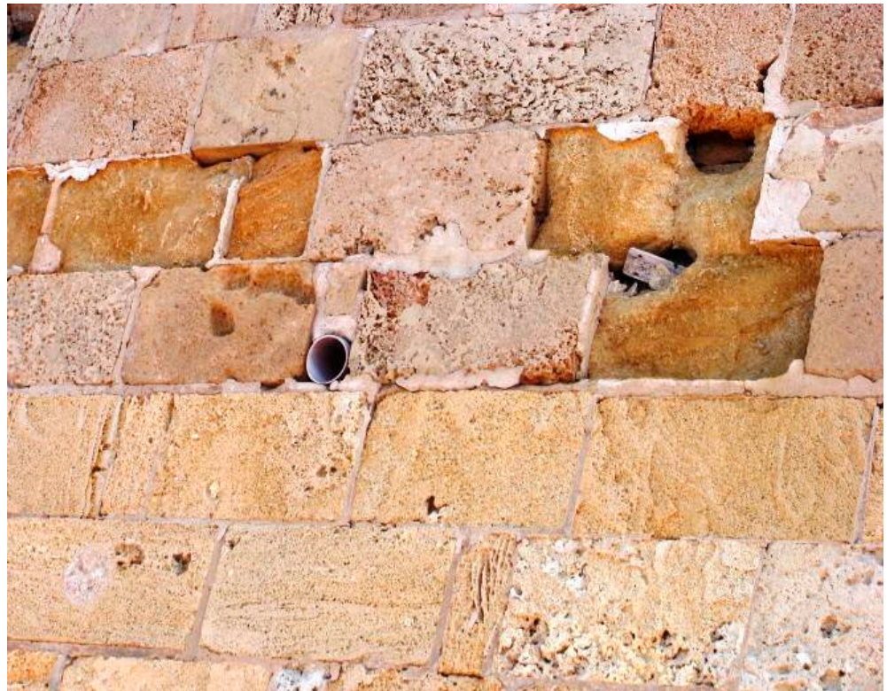
Figure 6. Back weathering of kurkar siding in the Panorama sea walls. Captured by the author on 27 November 2018.
