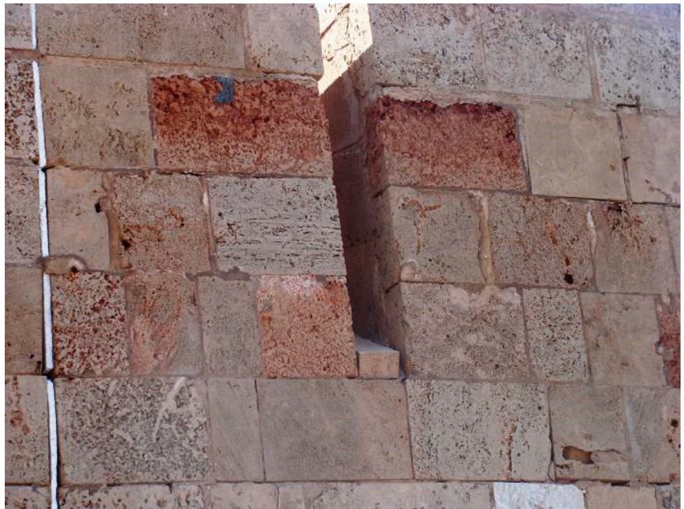
Figure 9. The coloration of kurkar siding in the Panorama sea walls. Captured by the author on 27 November 2018.
