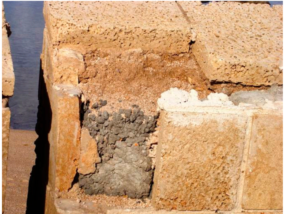
Figure 8. Break out of kurkar stone in the Panorama sea walls. Captured by the author on 27 November 2018.
