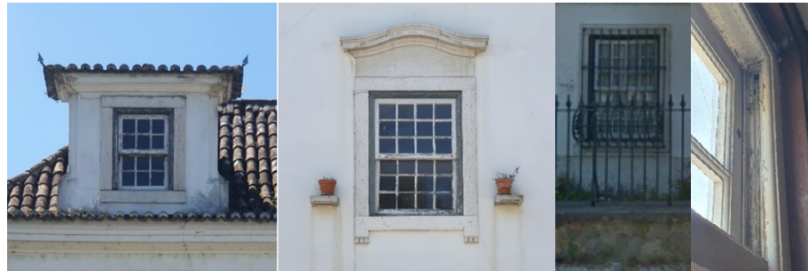
Figure 13. Distinct type of guillotine windows present in the main façade.
