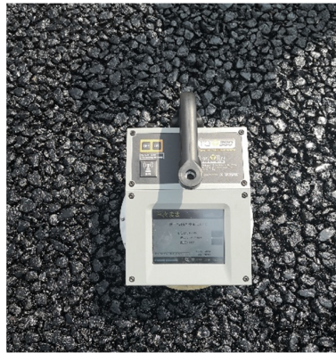
Figure 4. PQI380 used in in-situ test.
