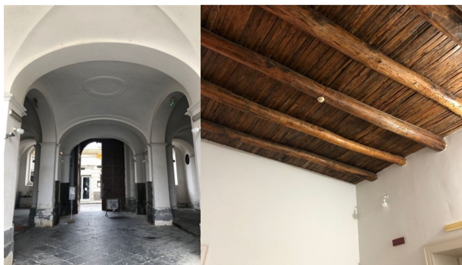
Figure 3. Internal areas Villa Vannucchi.
