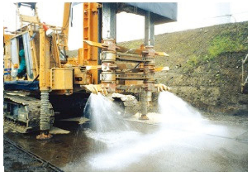
Figure 10. Mixing machine injecting atomized cement slurry [16].
