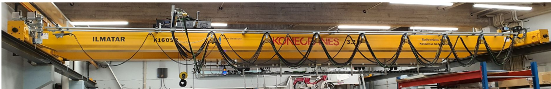
Figure 2. Overhead crane Ilmatar at Aalto University Industrial Internet Campus.
