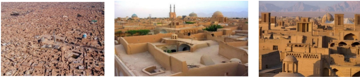
Figure 2. Various shots show details and components of the urban fabric of the old Yazd [33].
