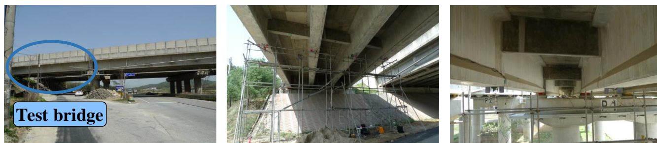
Figure 3. PSC I girder bridge.
