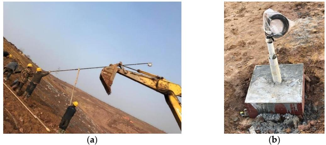
Figure 5. Bolt installation and concrete pile cap. (a) Bolt installation (b) Concrete pile cap.
