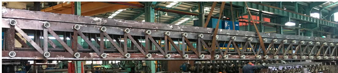
(a) EST composite girder at construction stage
