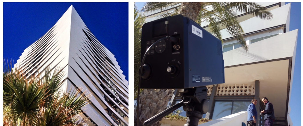
Figure 12. Measurement images of exterior finish plate.
