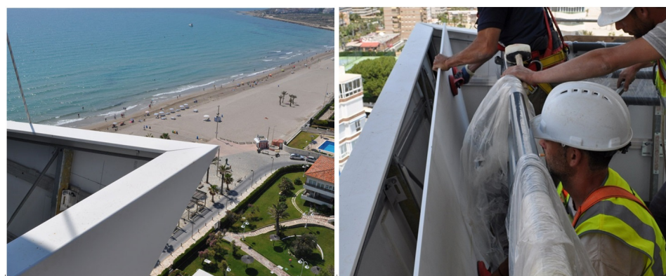
Figure 6. Images of interior and exterior finishing plate placement.
