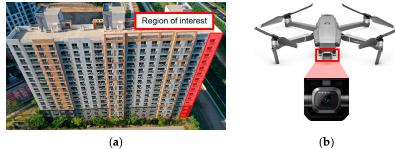
Figure 5. Experimental setup: (a) Front view of target structure with region of interest and (b) digital camera mounted-UAV.
