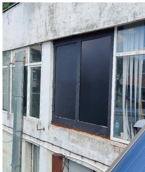
Figure 4. Building integrated Transpired Solar Air Collectors. TSC on the left and DSTSC on the right.
