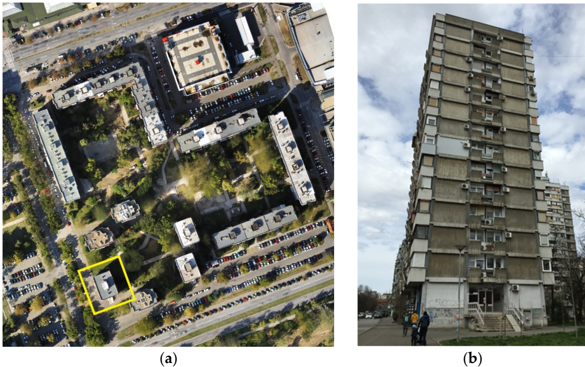
Figure 2. Residential high-rise building in Novi Sad. (a) Urban building block built in an industrial way in the second half of XX century with marked case study building; (b) high-rise residential building southeast façade.
