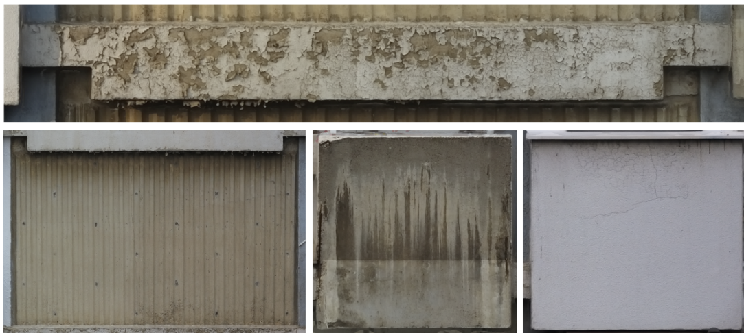
Figure 5. Realistic and clear presentation of façade elements on the generated orthofaçade image.
