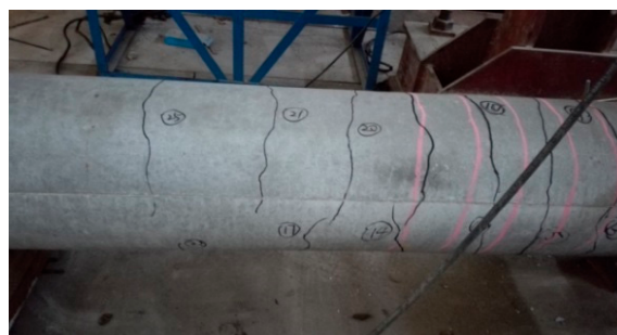
Figure 6. Some of the cracks generated in the PRC tube column specimen during loading.
