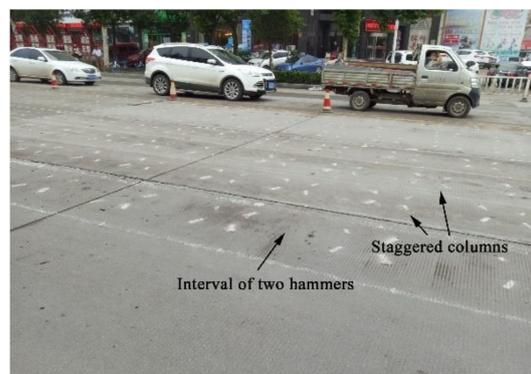
**Figure 17.** Crushing effect of interval two-step impacts.
