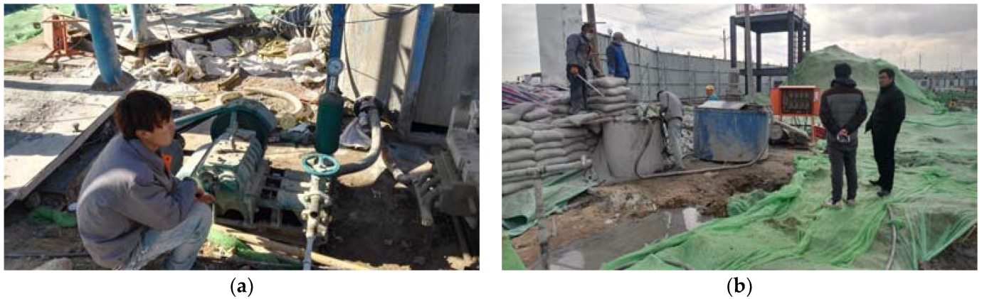
Figure 2. (a) Grouting devices; (b) Grouting volume and grouting pressure monitoring devices.
