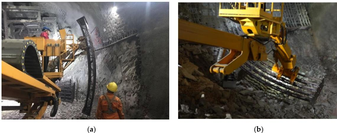
**Figure 26.** Mechanized installation of arch waist and inverted arch. (a) Arch waist and (b) inverted arch.
