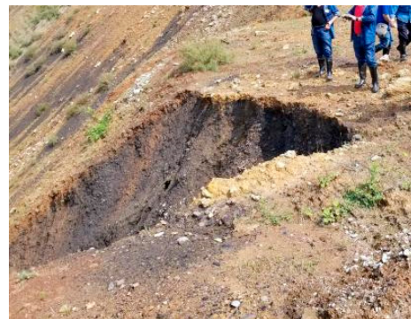
Figure 2. Status of No. 3 gully.
