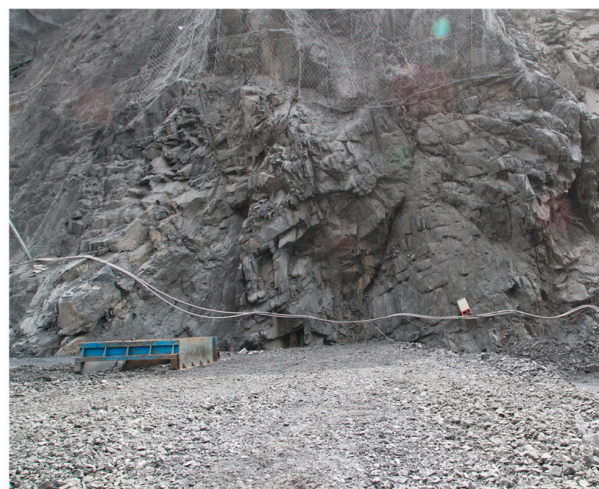
Figure 1. Slope rock mass of the left bank near the dam site of the Lianghekou Hydropower Station.
