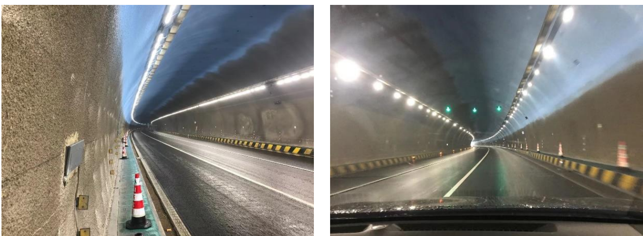
(a) Before the installation of al-foam board
