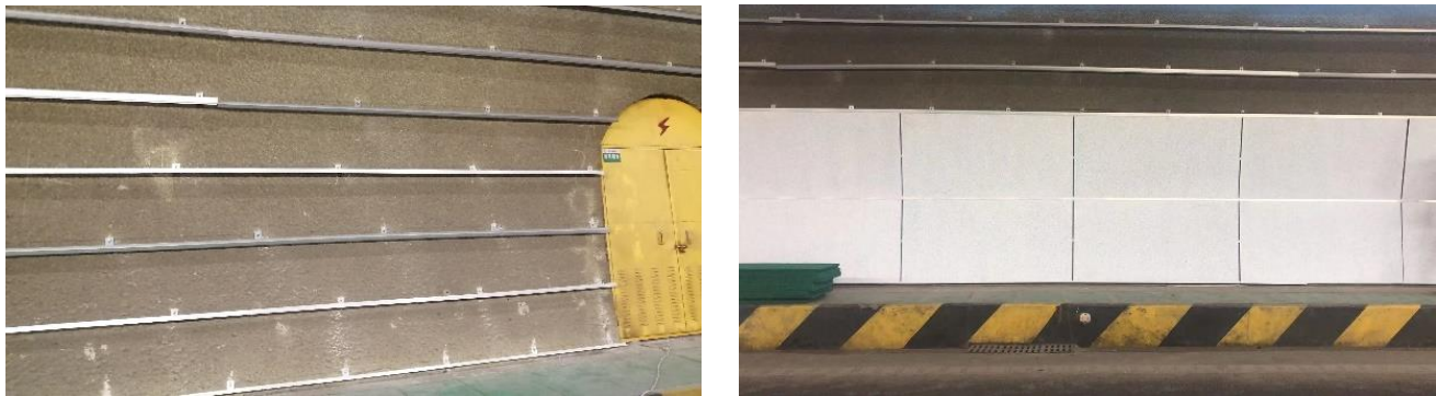
(b) During the installation of al-foam board
