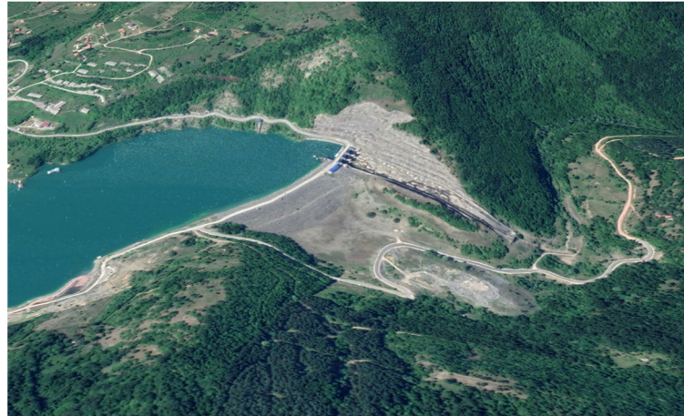
Figure 3. Zavoj dam—photo of the construction site.
