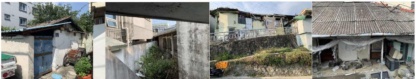
Figure 4. Status of vacant houses in residential areas.
