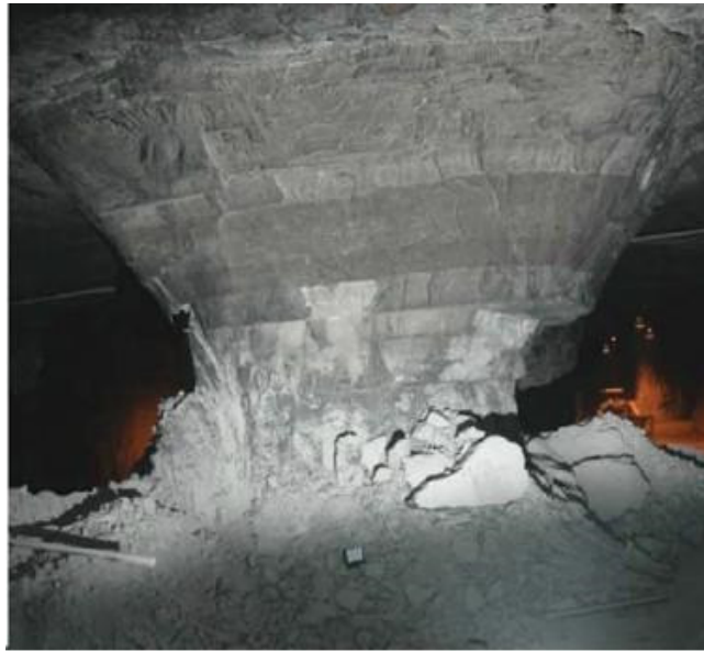
Figure 1. Joints with different inclinations in pillars [19].
