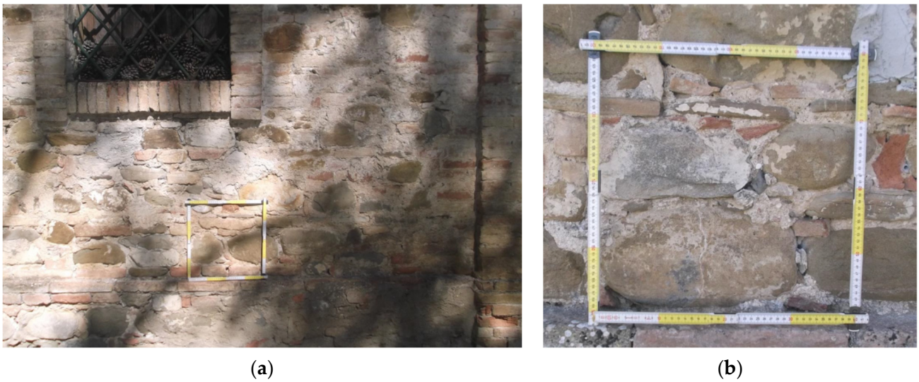
Figure 2. (a) Detail of the masonry walls of the building; (b) Masonry texture (inspection window dimension 40 × 40 cm).
