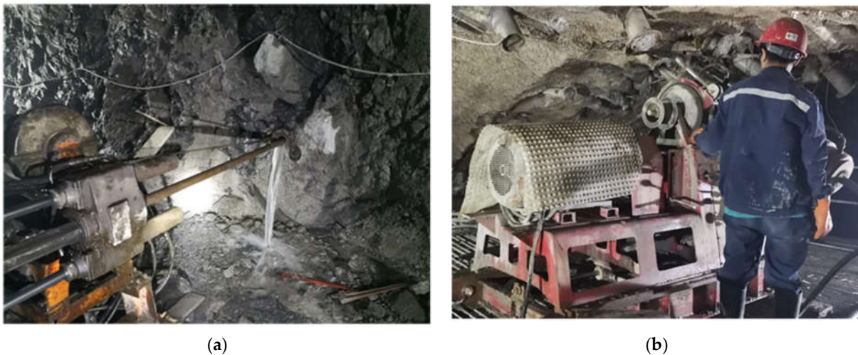
Figure 15. On-site diagnosis and treatment measures: (a) over-drilling. (b) grouting reinforcement.
