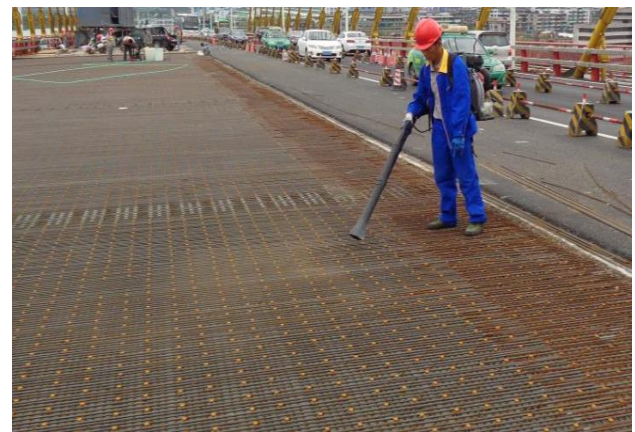
(b) Bridge deck cleaning
