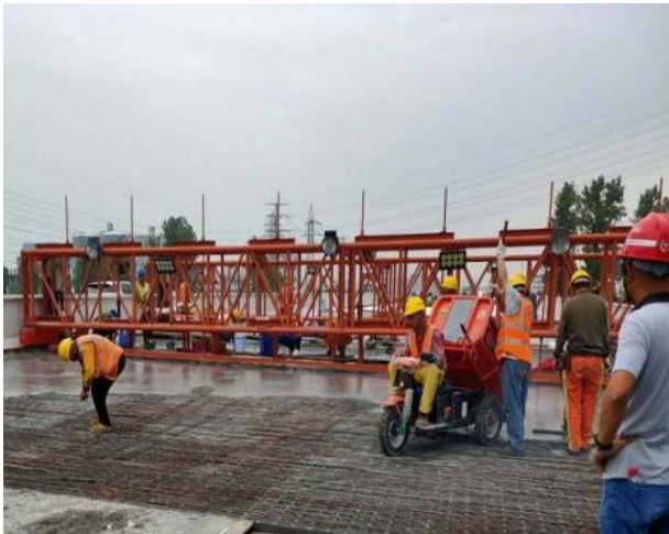
(a) Electric transport vehicle for pumping UHPC
