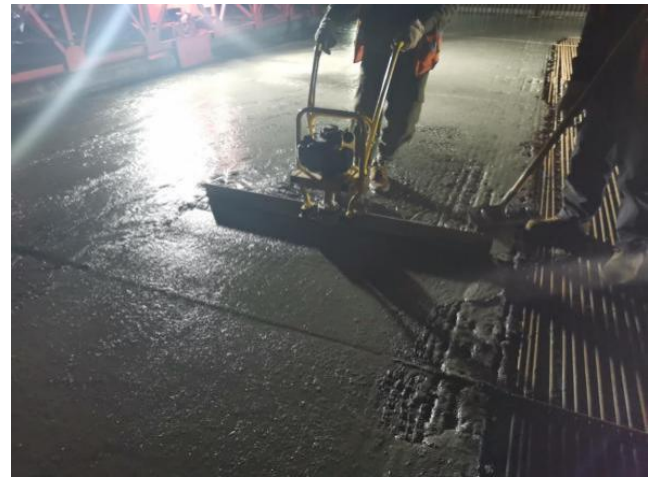
(b) Vibration construction with vibrating ruler
