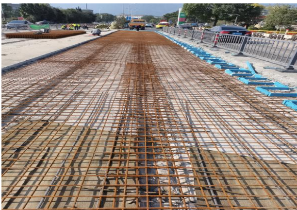
(a) Bridge deck rebar tying
