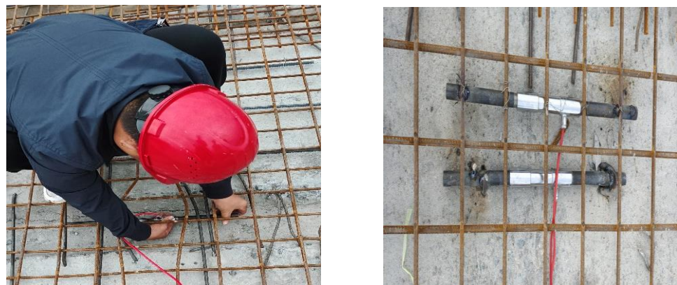
Figure 10. Gauge installation in the adhesion layer.
