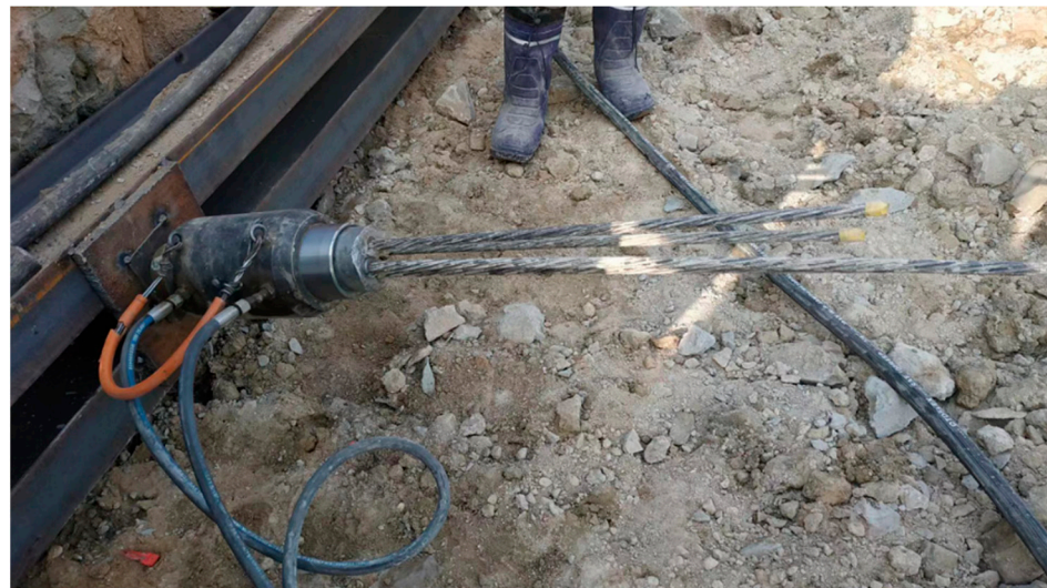
Figure 13. Tensioning of anchor cable.
