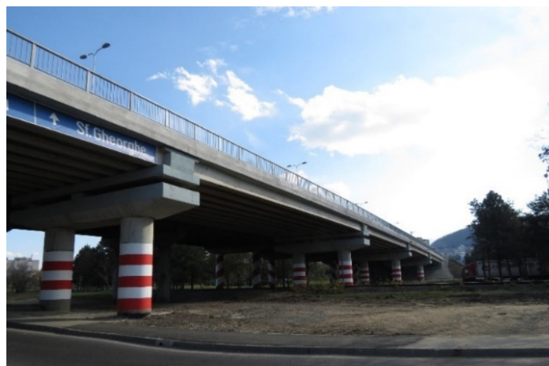
Figure 2. Fartec bridge in Brasov, Romania.
