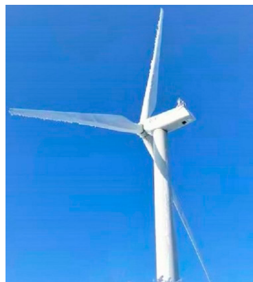
Figure 1. Icing on wind turbine blades.
