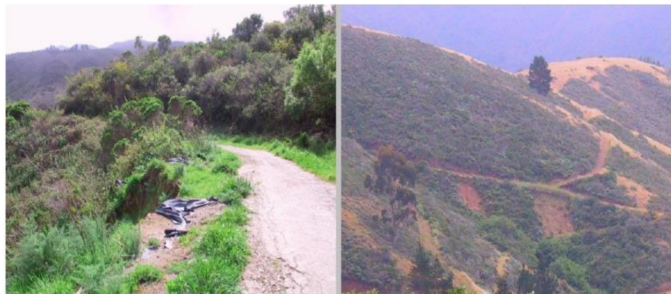
Figure 20. Rainfall-induced landslide in San Pedro Creek watershed [37].
