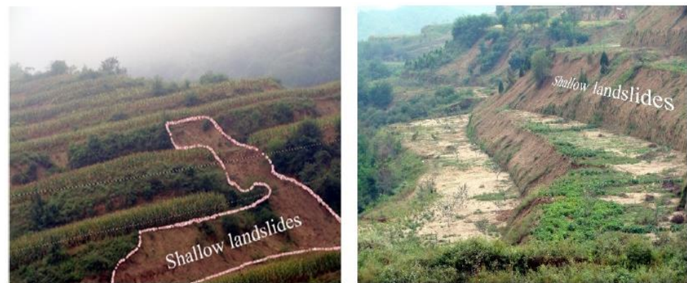
Figure 19. Shallow landslides in Yan'an China, July 2013 [128].
