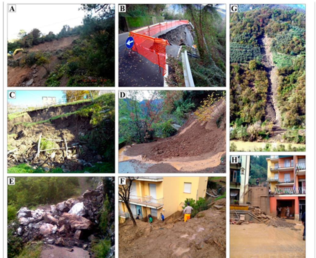
Figure 17. (A) Roto-translational slide; (B) Rotational slide cutting road downhill; (C) Landslide on terrace slides; (D) Uphill road cutting; (E) rockfall; (F,H) soil slip; (G) fast flow of earth [104].
