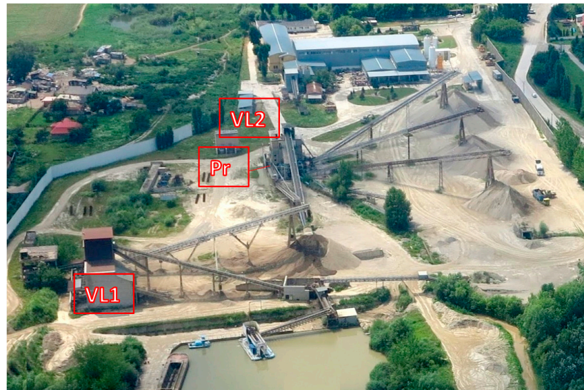
Figure 1. Sandy gravel production plant.
