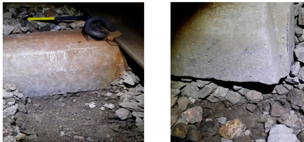
Figure 2. Damaged ballast.
