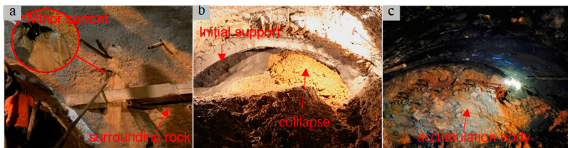
Figure 10. Distinctive actual disaster processes. (a) Minor current; (b) collapse; (c) accumulation body.
