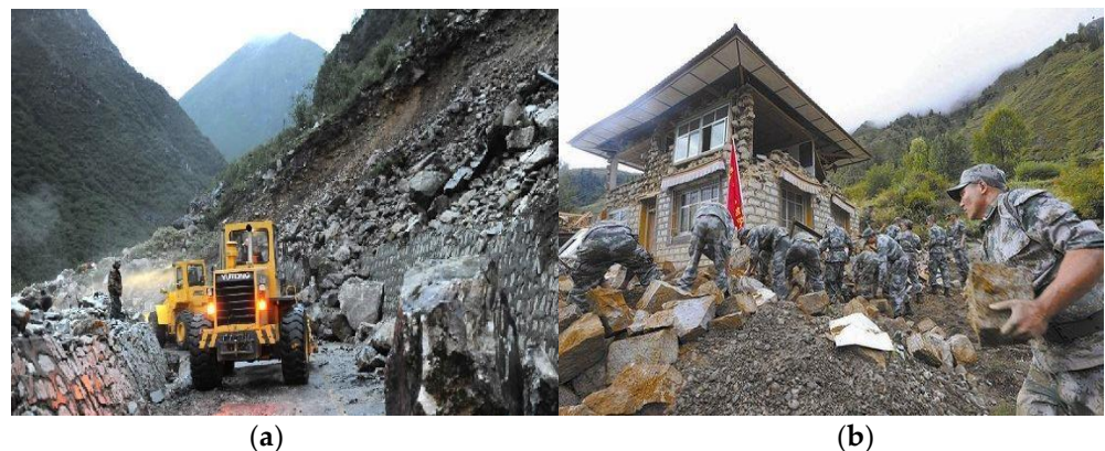
Figure 2. The Sikkim earthquake triggered landslides in Yadong County: (a) S204 road was interrupted; (b) houses collapsed.
