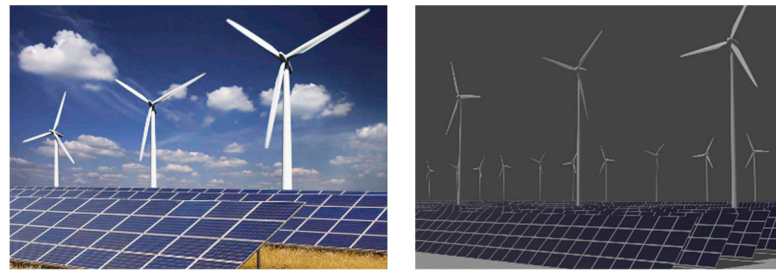
Figure 9. Digital twin of wind and PV plants. The left image shows the wind and PV power generation equipment in real space, while the right image shows the corresponding digital twin 3D model of the equipment.
