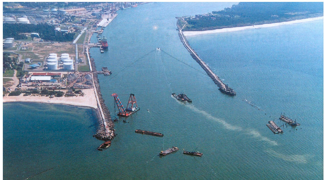
Figure 1. Klaipeda port gates renovation process [10].
