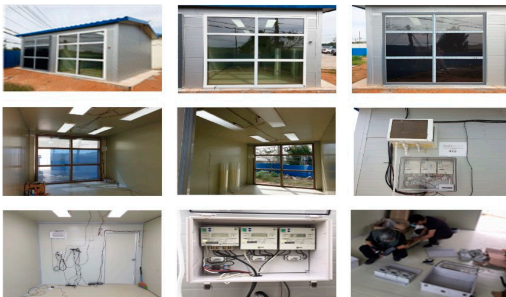
Figure 9. Construction of test and reference rooms.
