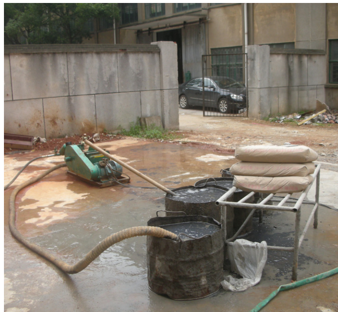
Figure 2. The grouting system.
