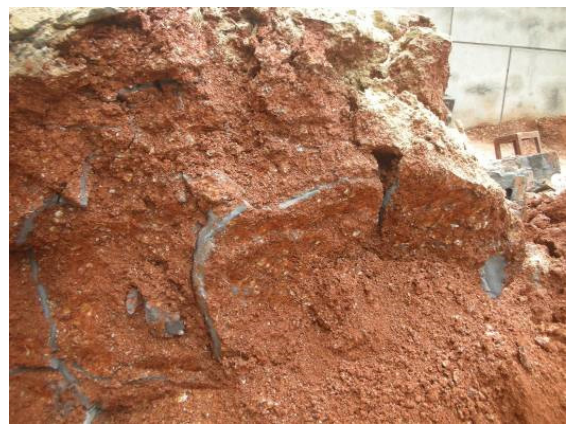
(b) grouting in clay and silty sand filling zone.
