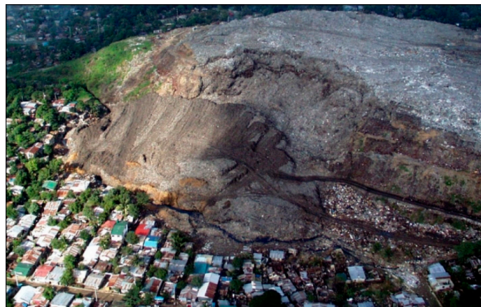
Figure 1. Slope failure in the Payatas landfill in Quezon City, Philippines (source: International Journal of Geoenvironment Case Histories).
