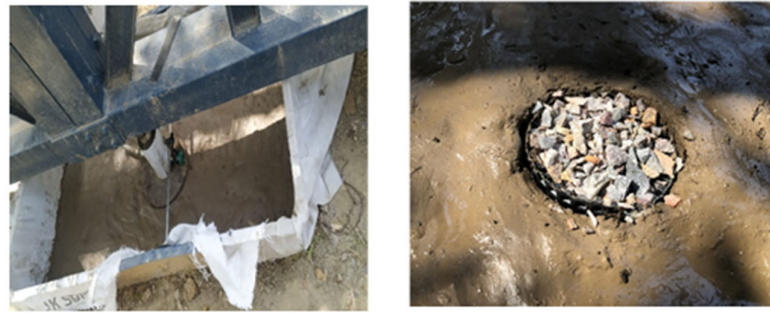
Figure 2. Test tank and stone column installed and reinforced with geosynthetics.
