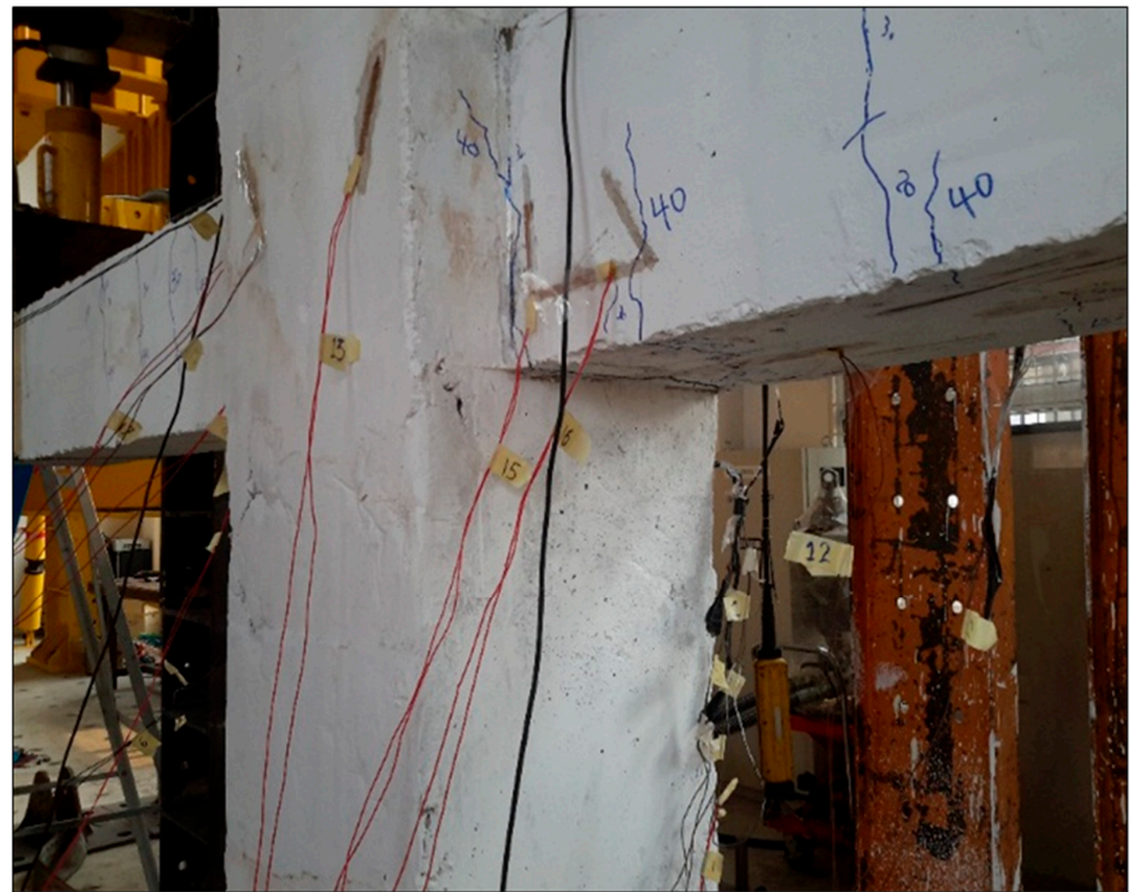
(a) Crack pattern in CS1
