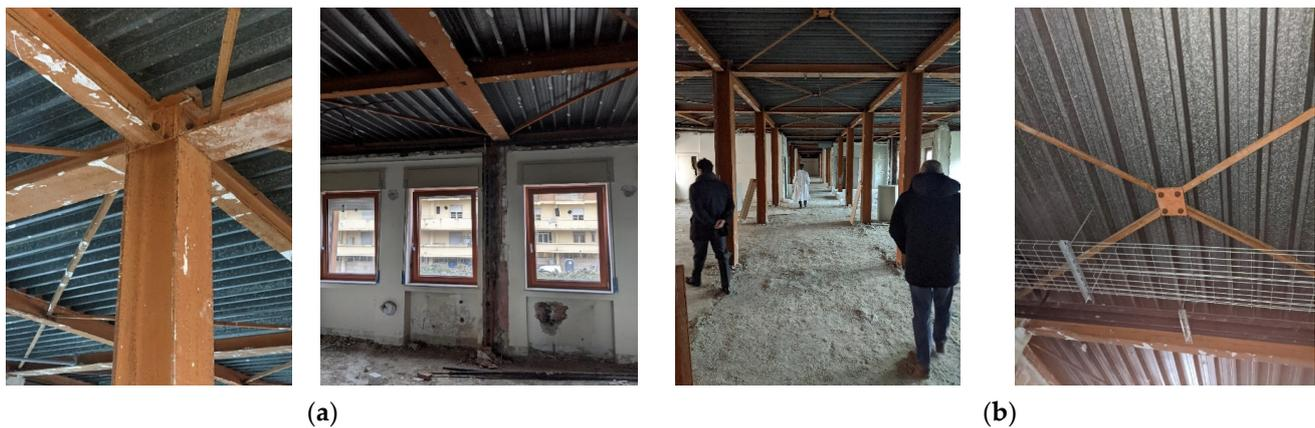
**Figure 4.** Construction details: bolted connections between columns and beams (a); horizontal concentrically bracing system (b).
