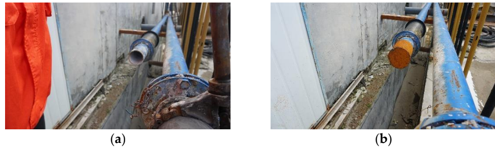
Figure 7. Schematic diagram of the pipeline before and after damp (a) Undamaged pipeline (b) damaged pipeline.
