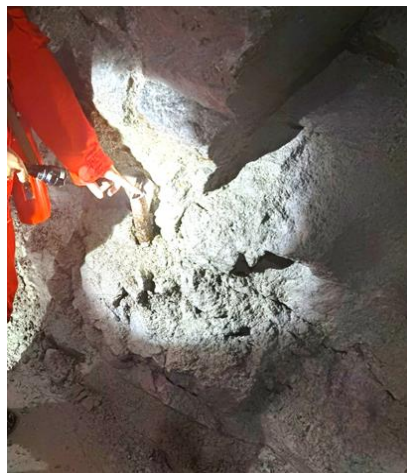
Figure 2. The layered subsidence problem was observed from the adjacent mine room.
