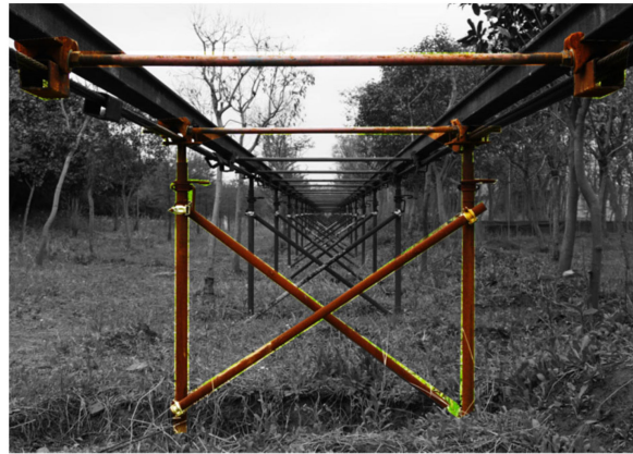
Figure 5. AERORail structure and support picture.
